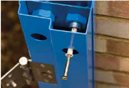
STEP 4: Insert the frame fixers.
